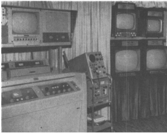
Fig. 1. Demonstration setup for interswitch operation on two television standards
