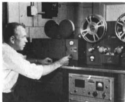
Fig. 4. Re-recording from 35mm magnetic film to 16mm negative soundtrack.
