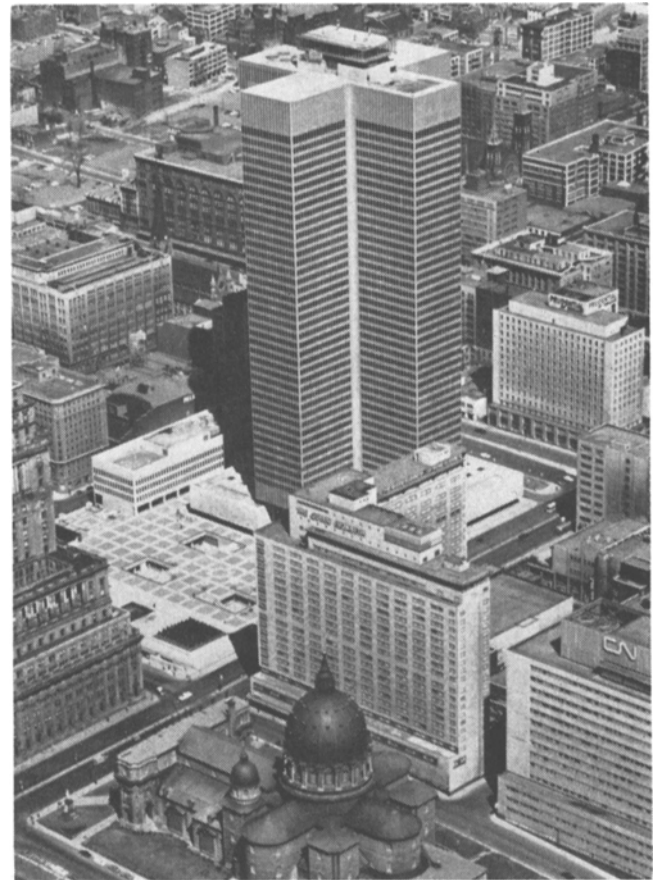
The Place Ville Marie , a new cruciform building in downtown Montreal, looms above the Queen Elizabeth Hotel, site of the 98th SMPTE Conference.
