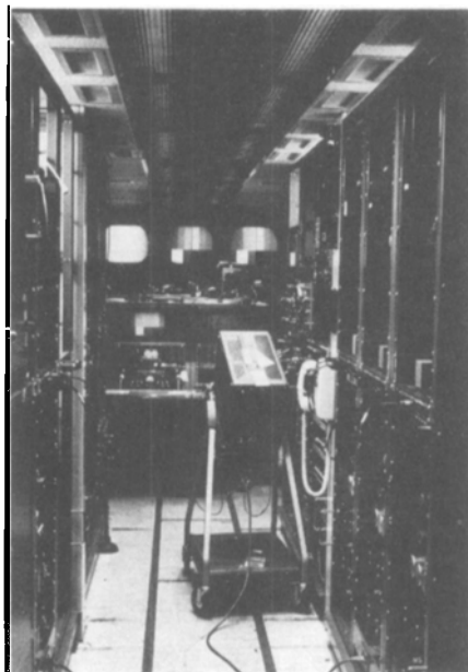
Fig. 3. Looking toward the front of the A unit.
