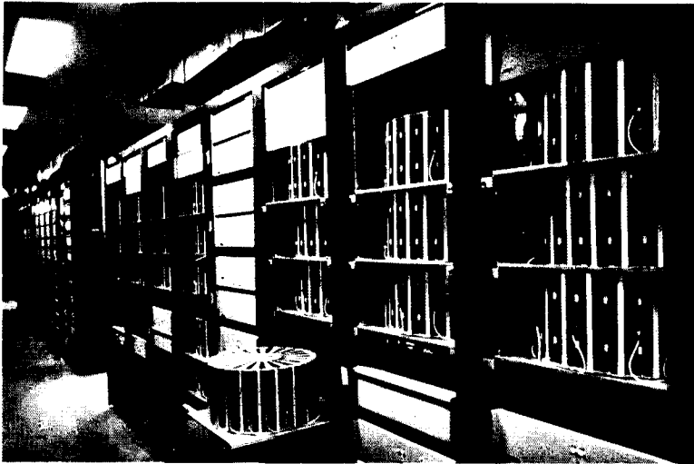
Fig. 2. Program Switcher: Shows approximately half of the Program Switcher, with video racks in the foreground, audio section at left.
