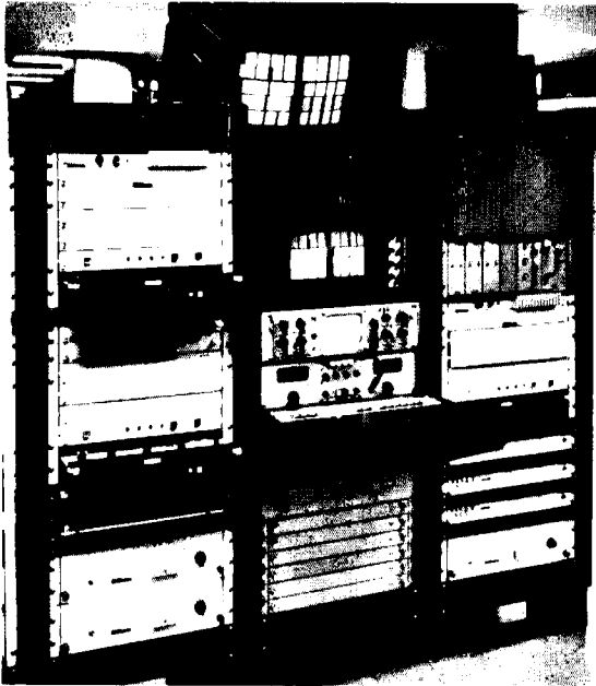
Fig. 9. Live Camera CCU group; shown are three CCUs grouped with monitoring.
