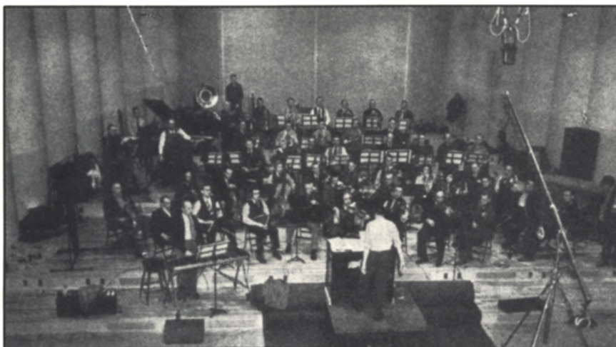
Scene on orchestra stage, showing convolutions of orchestra shell designed to improve acoustics • The New Walt Disney Studio • W. E. Garity and J. L. Ledeen • JSMPE , January 1941
