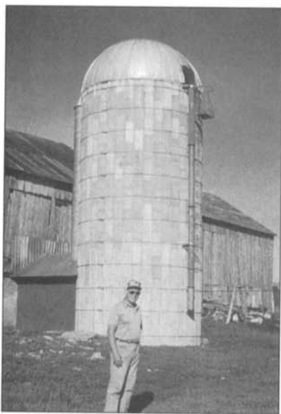
A view of Kenbar Farm.
