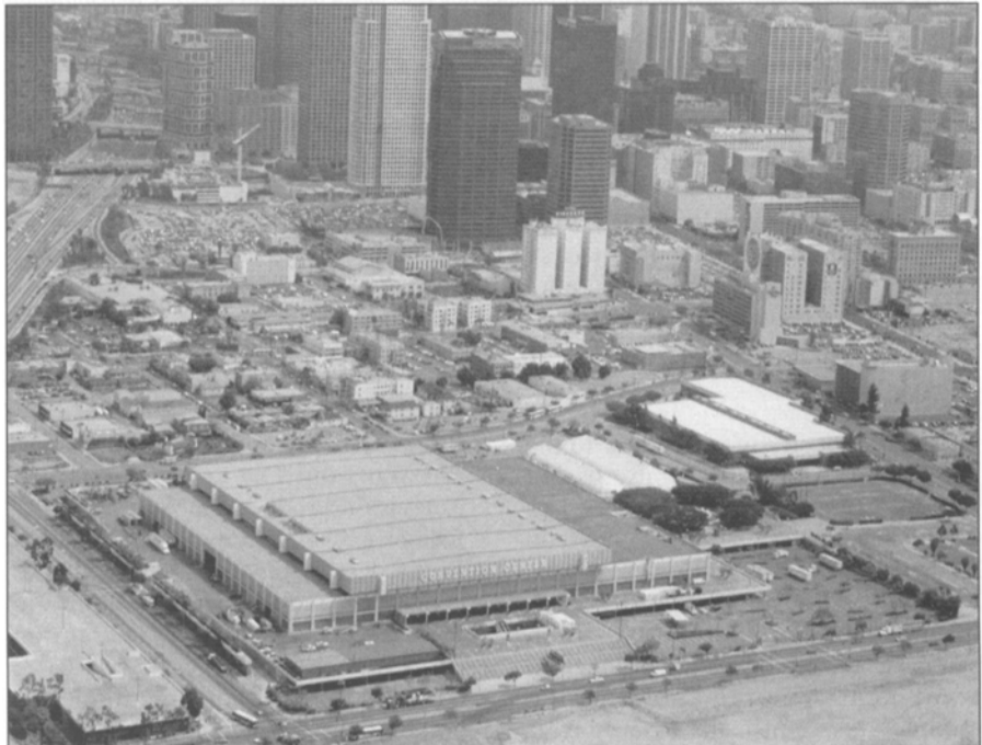
An aerial view of the Los Angeles Convention Center.
