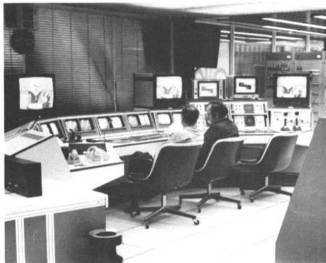
Figure AR-1. Central control room in new Television Center.
