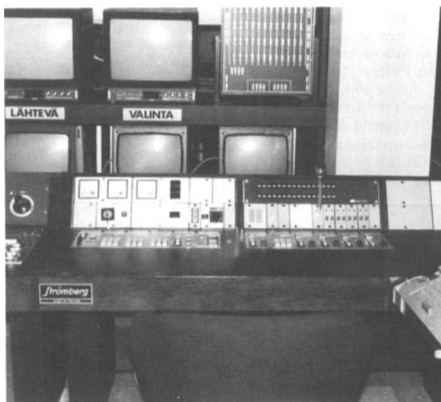
Figure F-3. Strömberg Novalit lighting control equipment in the news studio.
