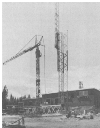
Figure F-3. The Tampere mast under construction.
