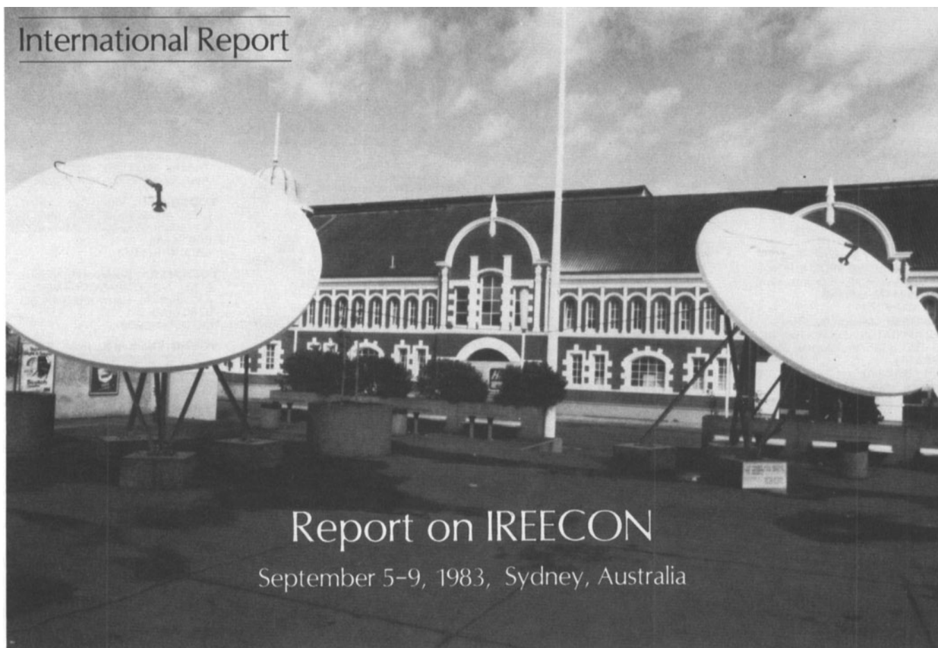
A pair of co-phased 4.5-m receive-only satellite antennas were set up adjacent to the IREECON exhibition building at the Sydney Showgrounds.
