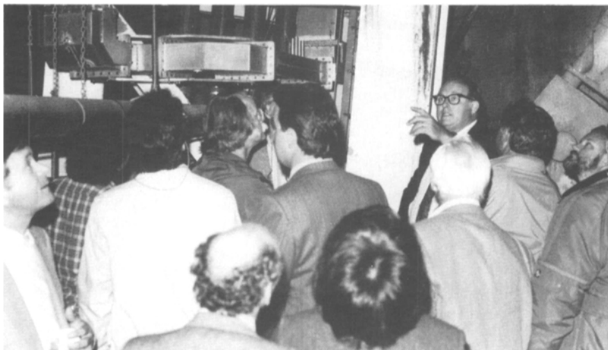
Attendees at the August 28 San Francisco Section meeting tour the equipment building at the base of the Sutro Tower, with Don Lincoln providing comments and information.
