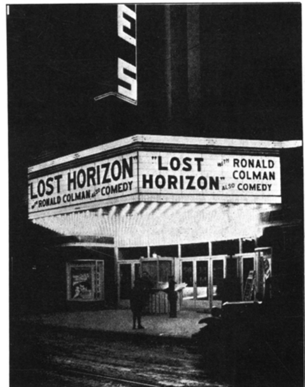
Changeable-letter sign with extended background to allow use of letters of a variety of sizes • Progress in Motion Picture Industry • Report of the Progress Committee • JSMPE, August 1938.
