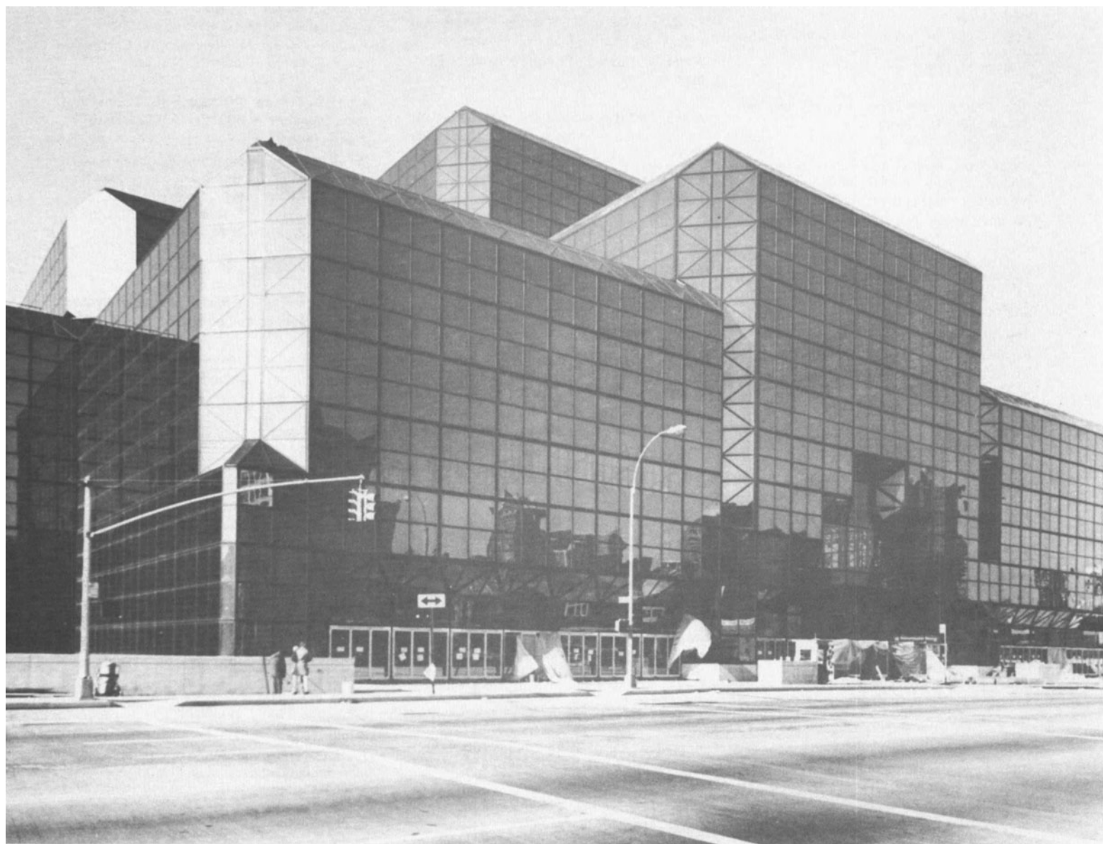
The Jacob K. Javits Convention Center, site of the 132nd SMPTE Technical Conference and Equipment Exhibit.
