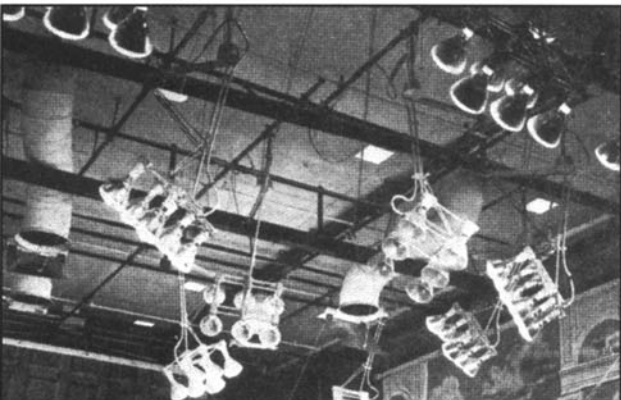
(Left) Set of remotely controlled units, with hemisphere of operation tangent to each other; (Right) Light-control bridge • Remote Control Television Lighting • W. C. Eddy JSMPE, September 1940.
