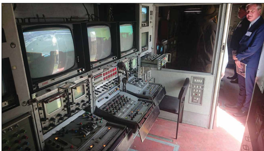
Monitoring was done by humans watching oscilloscopes. No automated quality control.
